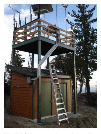
The MHRC Repeater is in excellent working order. We (the MHRC) perform monthly inspections to the site. We check and monitor the Solar Charge output, Battery condition, Antennas, Cables and overall facility inspection.
