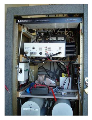
The photo above is a look into the MHRC Repeater cabinet. It contains a controller, radio, charge controller, power supply, tuned cavities and a 250 pound 12 volt battery.
